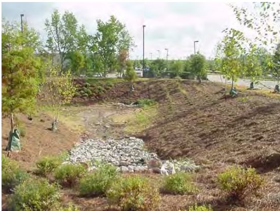
Picture 1: Dry extended detention basin
