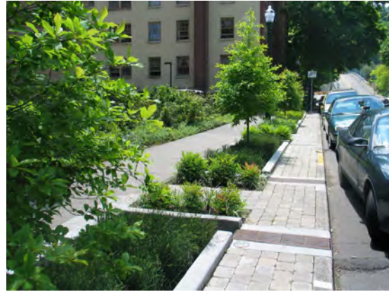
Picture 2: Bioretention planters
