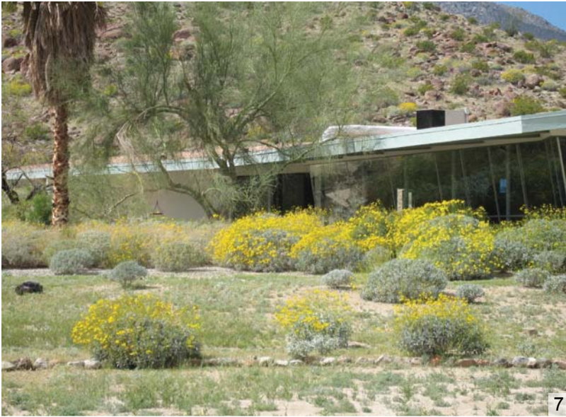
View of the Desert Research Center, surrounding landscape and hillside to the northeast
