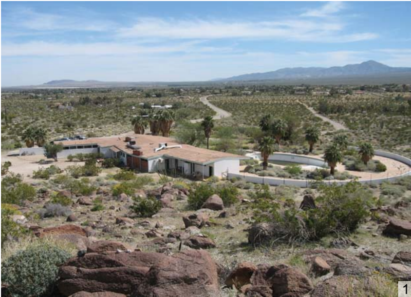
1 View looking southeast from adjacent hillside towards the Desert Research Center
