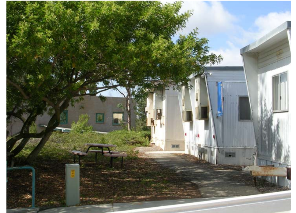
View northwest, from west/center of site, at old trailers and adjacent courtyard in northwestern corner of site. Humanities Office Building is in background.
