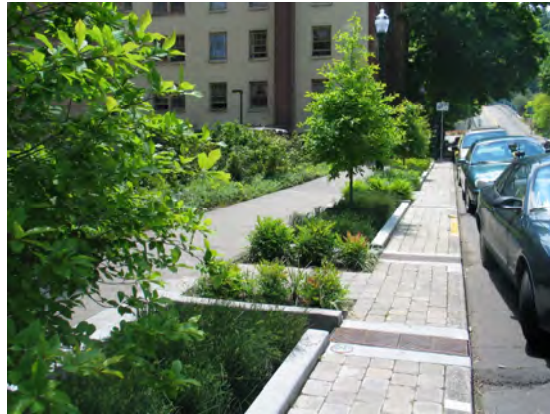
Picture 1: Bioretention planters
