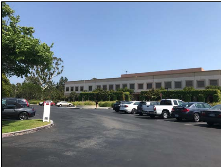
View 3: Southwest corner of the project site looking southeast toward MSTB.
