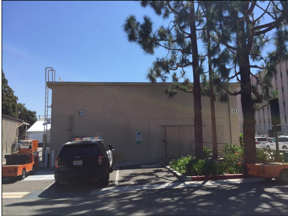
View 5: View from western boundary of project site looking east toward project site.
