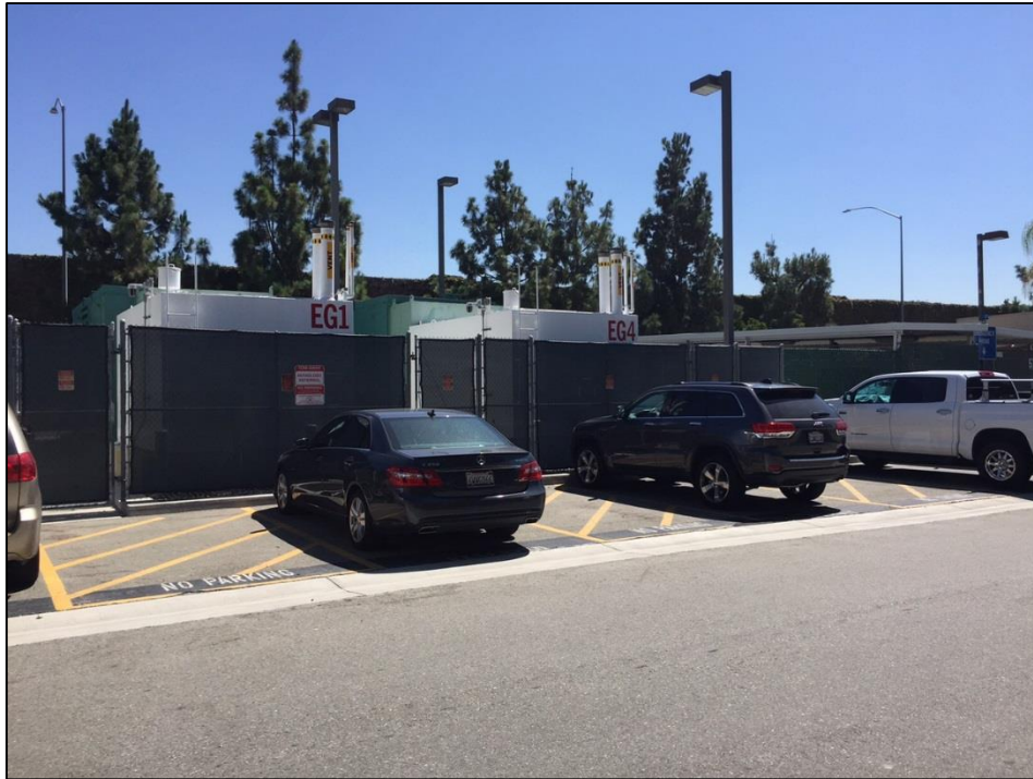
View 5: View from southwest corner of project site looking east toward the project site.
