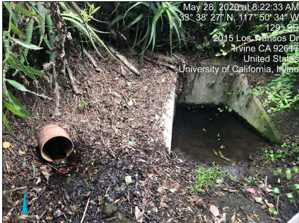
Upstream stormdrain inlets into the drainage.
