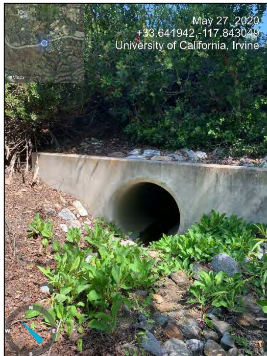
Downstream drainage outlet with yerba mansa.
