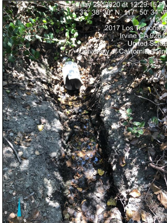
Existing storm drain inlet located on the downstream end of the drainage.
