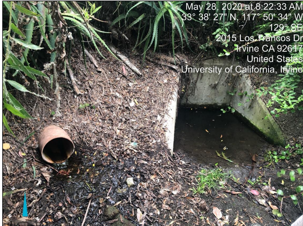
Upstream stormdrain inlets into the drainage.
