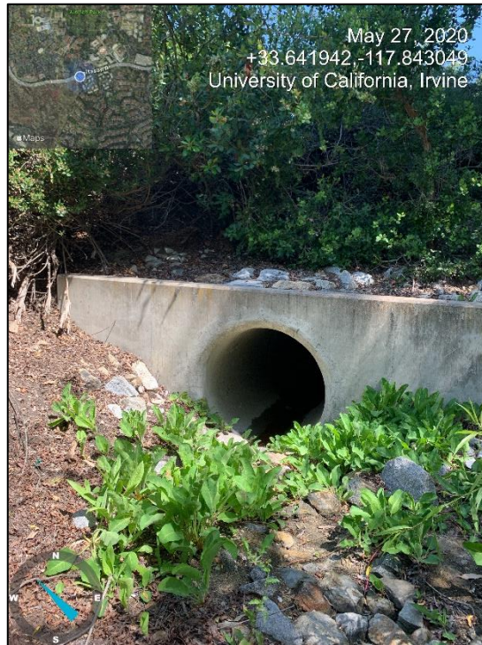
Downstream drainage outlet with yerba mansa.
